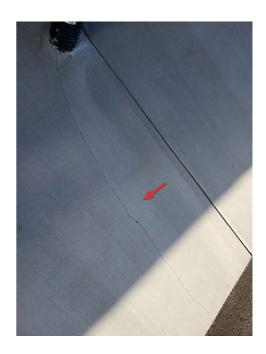
3.4.1 Eaves, Soffits & Fascia **OBSETVED CRACK IN SOFFITS** Recommendation Recommend monitoring.
